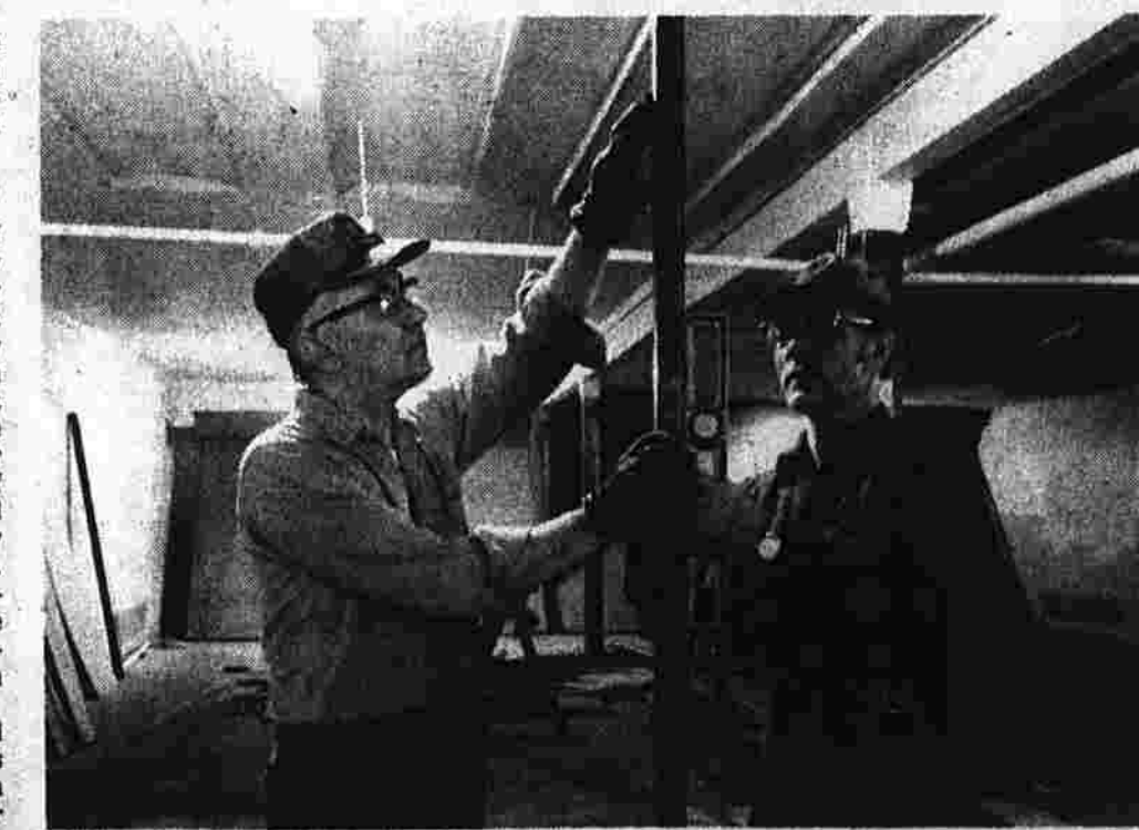
Constructing Rifle Range
